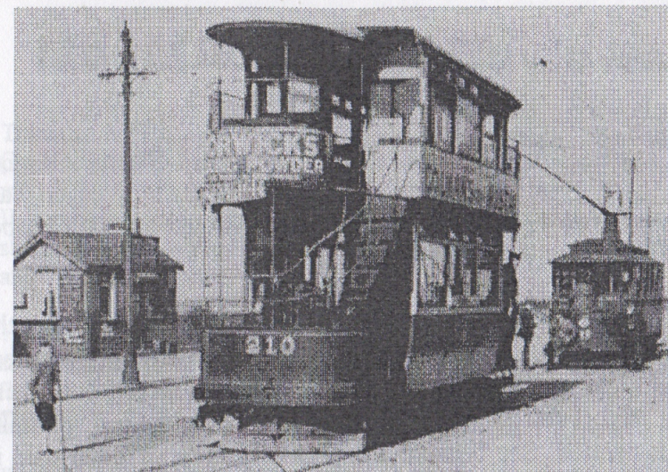
Car 210 shows the typical appearance of the 20 Dick Kerr cable cars after 1907 when top covers were fitted. Note the half balcony effect left by the open stair design.
